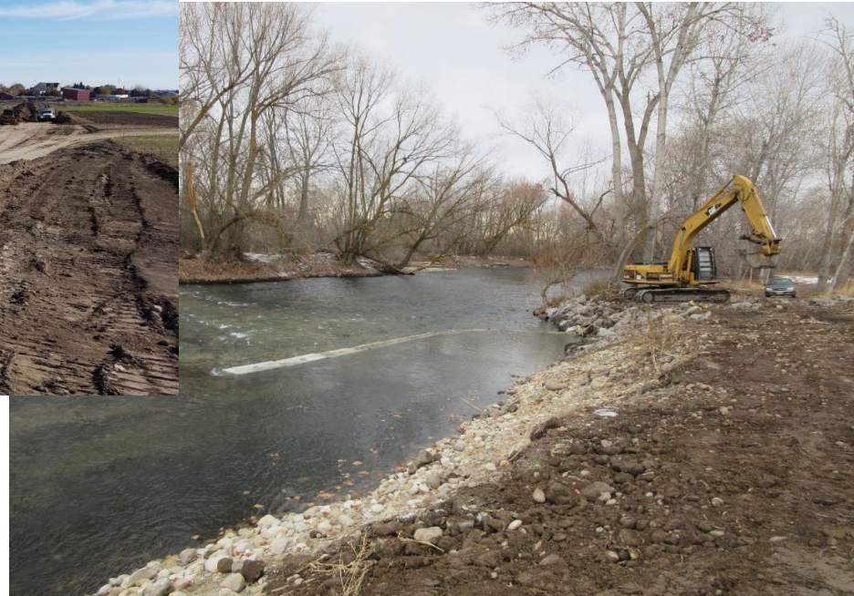
Bank stabilization on Boise River
