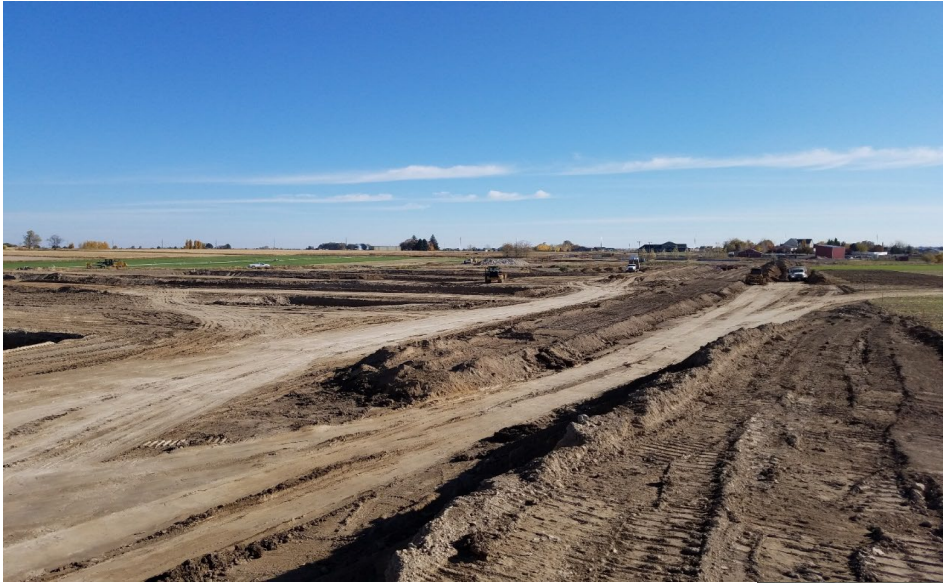
Construction of flood retention pond near Twin Falls
