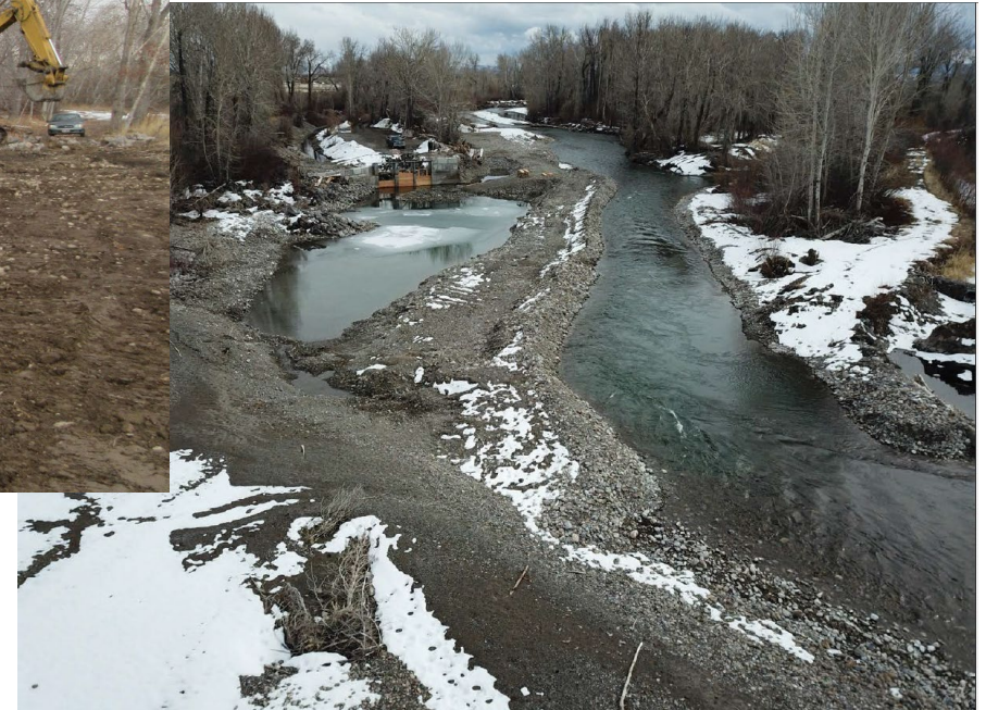
Channel reconstruction on Big Wood River
