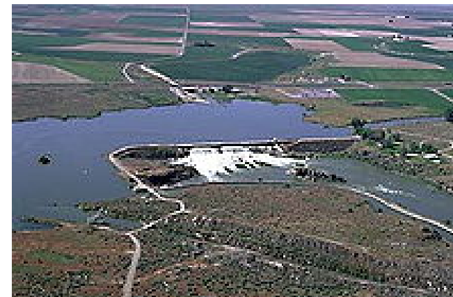
Milner Dam – Lower end of WD01
