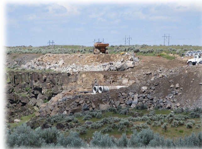
Construction on the Wilson Canyon Recharge Site
