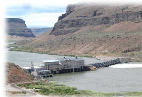
Swan Falls Dam
