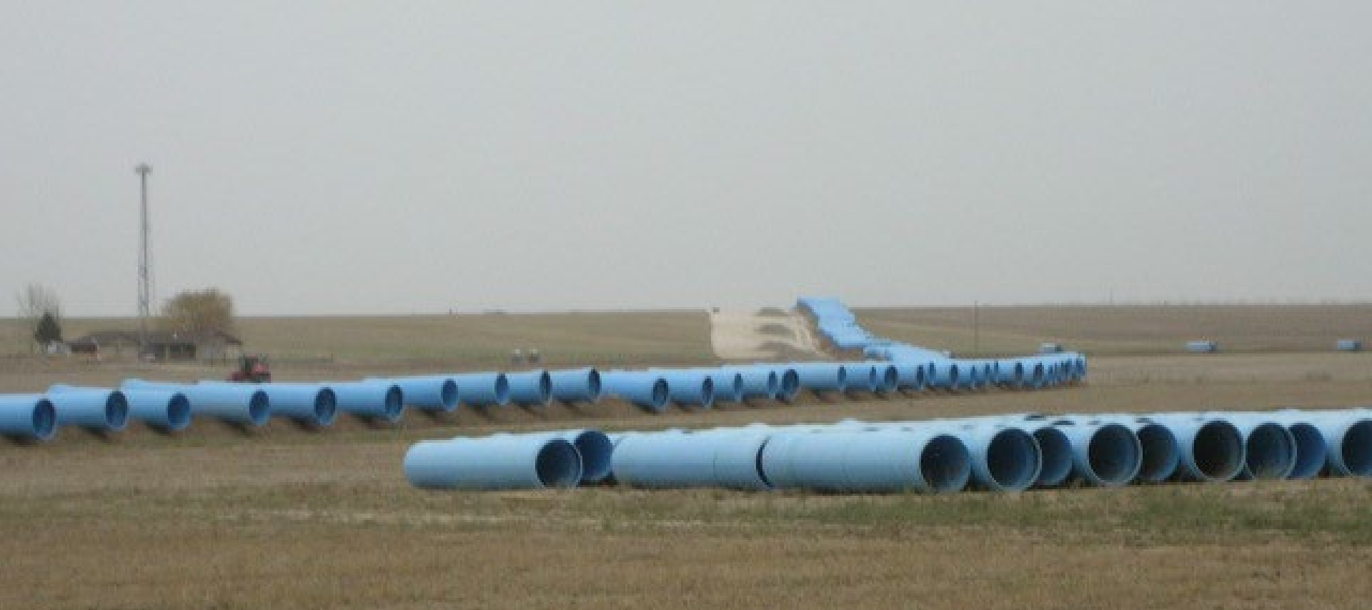
54-inch Pipe Staged Along the Route
