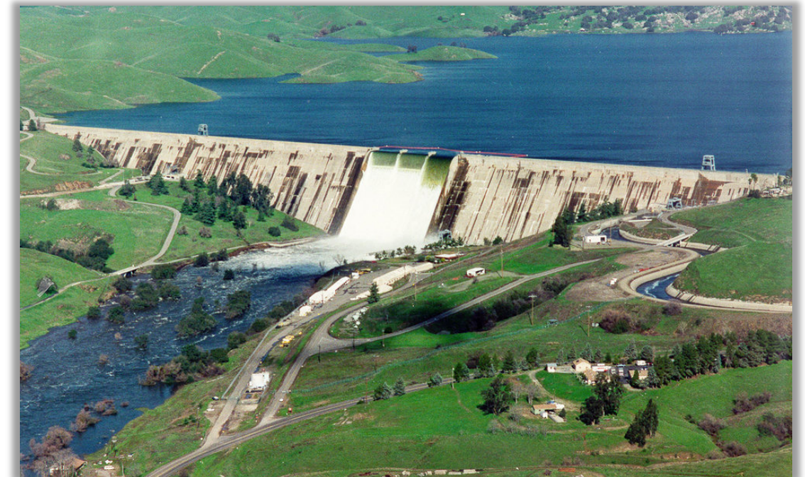
Friant Dam and Millerton Lake from Friant Water Authority
