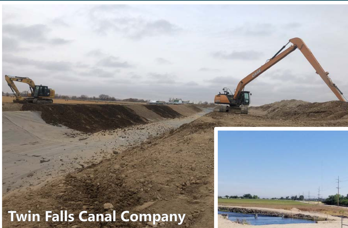
Geomembrane liner on 4,200 feet of the High Line Canal ($239,000 WaterSMART grant)
