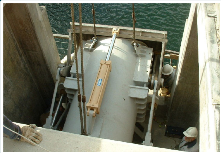
February 2003 Clamshell gates being installed
