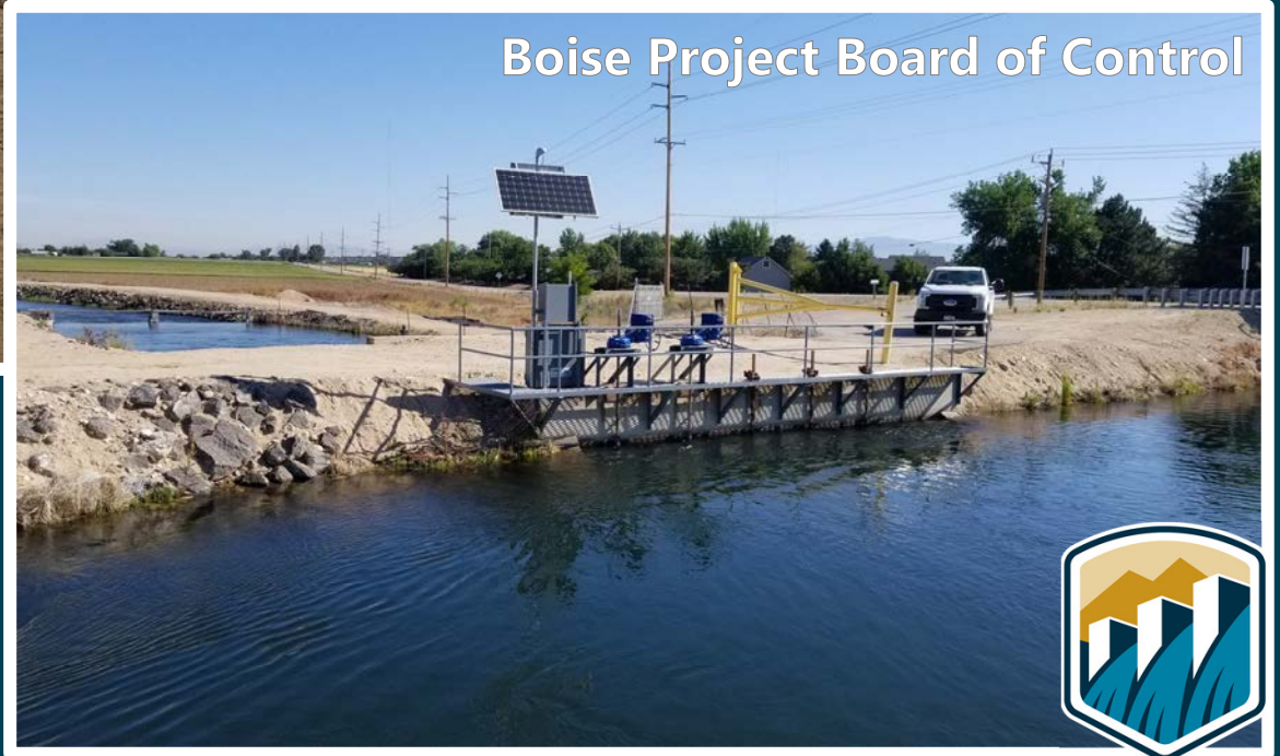
Rawson automated headgates installed on the New York Canal ($31,425 WaterSMART grant)
