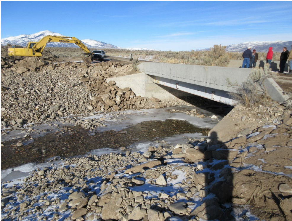
West bridge abutment rip rap installation
