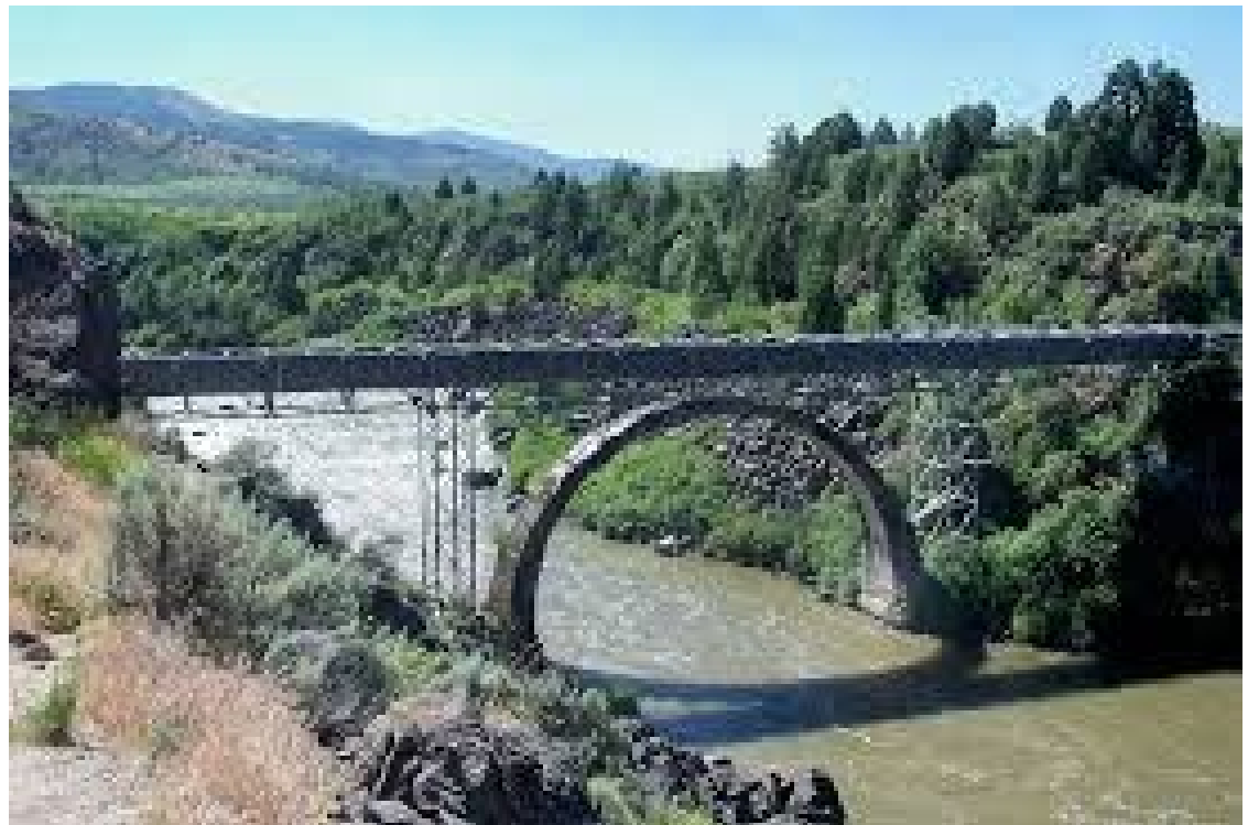
Last Chance Canal Company flume over Bear River
