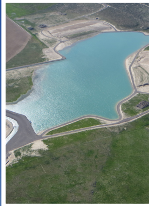
Kinyon Pond Re-Regulation Reservoir
