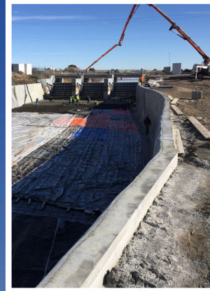
Canal Lining below Headworks at Milner Dam
